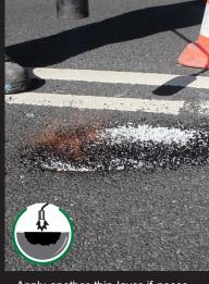
Apply another thin layer if necessary. Finish by sprinkling anti-skid aggregates on the hot material
