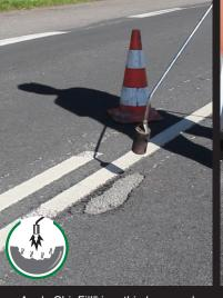
Apply ChipFill® in a thin layer and spread out (maximum 15 mm thick)
